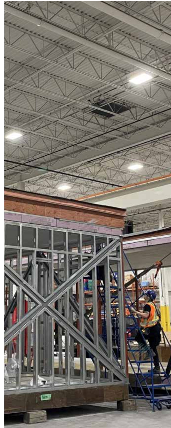
Modular construction in progress at Fero's facility in Stoney Creek, Ontario.
